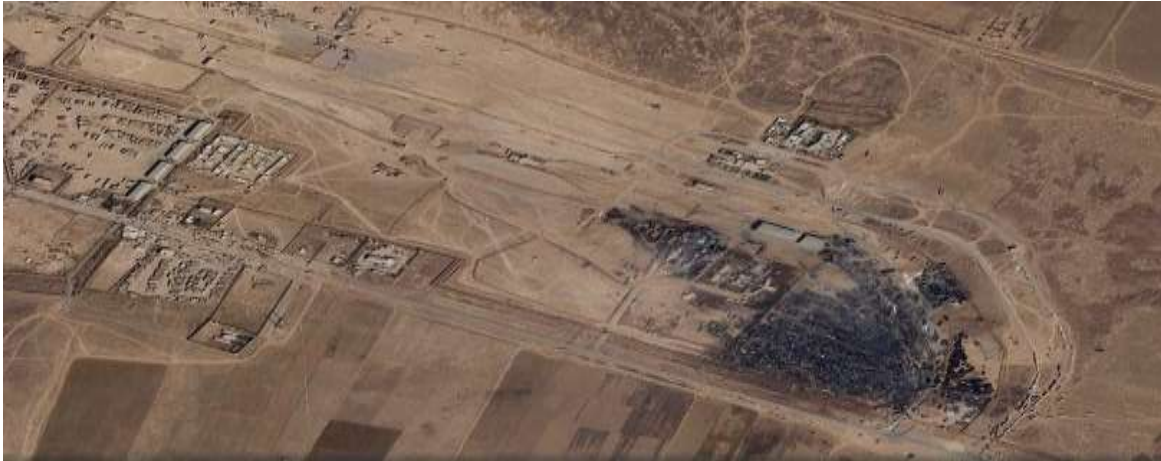
(An image of destruction caused by the fire incident in Islam Qala port)
